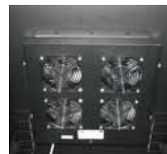
Image shows roof mounted Smart Net Fan Unit fitted in cabinet.
